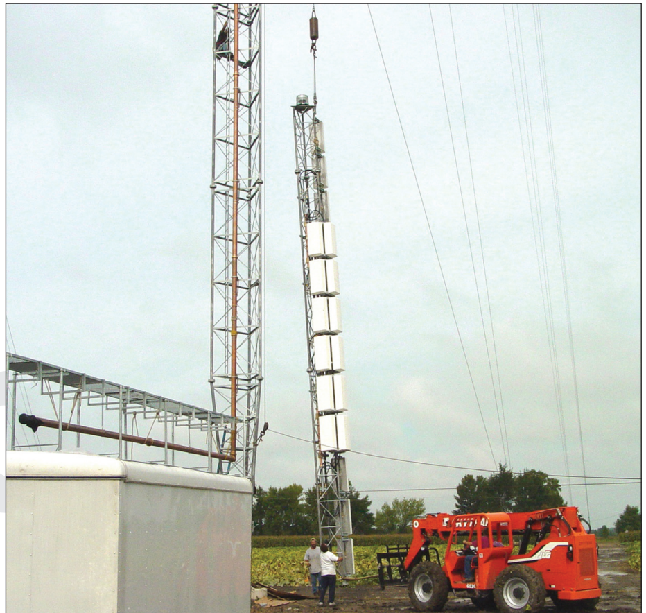
The WBSF Channel 46 PSI antenna is hoisted into place.
